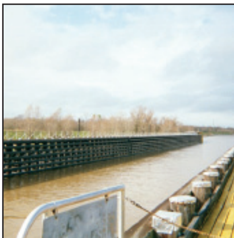
Intracoastal waterway guidewall
