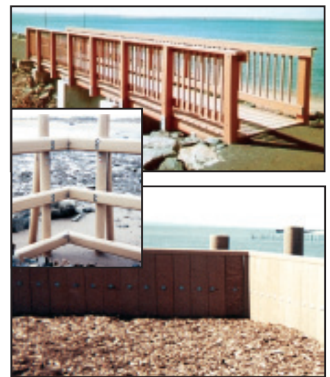
Retaining wall and pedestrian bridge
