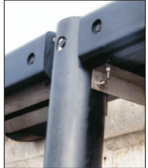
Closeup detail of fender pile and wales
