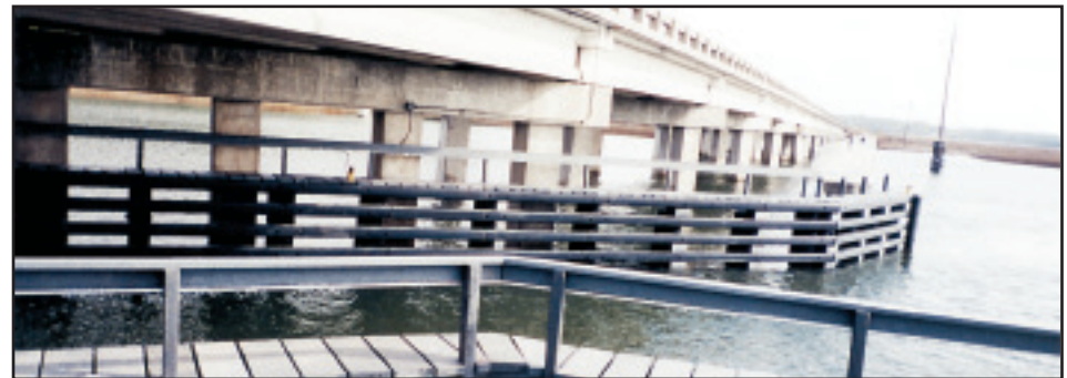
Bridge Pier Protection
