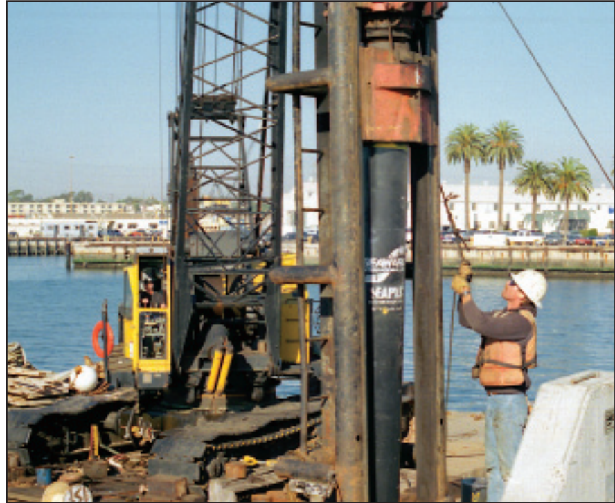
SEAPILE Composite Marine Piling being installed
